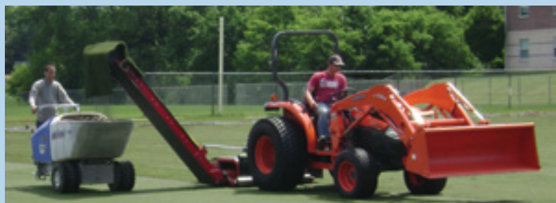
Removing infill
